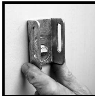
Turn the U-Clip™ until it is flush with the insulation
