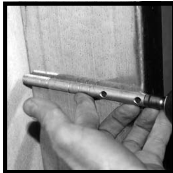
From the inside of the building, drill thru the sheathing
