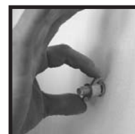
5. Hand tighten Wing Nut™ until washer dimples into the insulation
