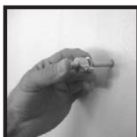
2. Push screw into insulation as far as possible with your hand
